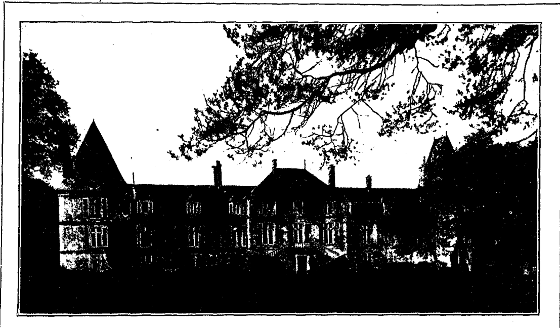
LE CHATEAU (XVII CENTURY), VAUXBOIN, AISNE. USED AS A HOSPITAL BY F.F.N.C. SISTERS, NOW IN RUINS.
